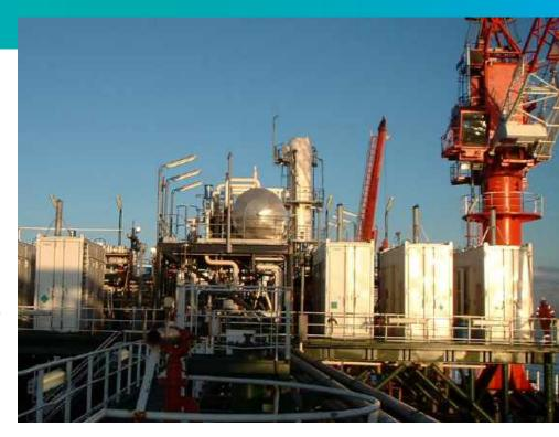
way to design the package as separate sub-assemblies, each weighing no more than 3.5 tons. This made it feasible to carry each assembly by helicopter and assemble it on site. "Without our 3D design and analysis capability, this project would have taken much longer," says Peter Elliott-Moore, engineering director at Calder.
